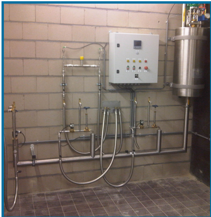
Filling point: un-insulated valves & Phase Separator for open & closed dewars
