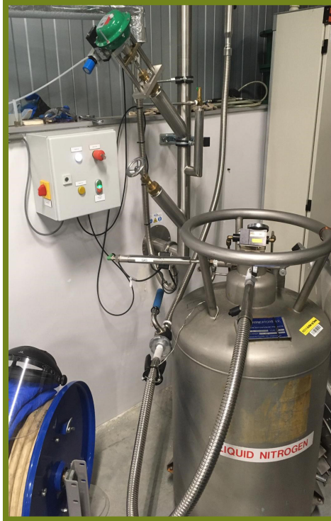
Filling point: vacuum insulated
