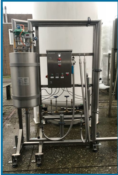
Filling station with uninsulated valves
