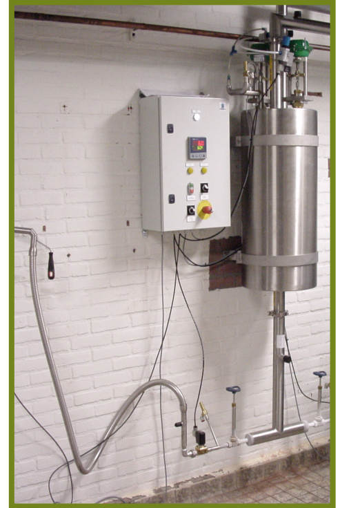
Filling point: un-insulated valves & Phase Separator
